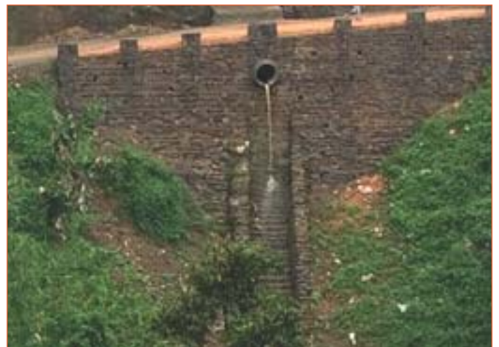
Figure 4: CRSM Retaining wall and providing of Hume pipe culvert at Mon Town
