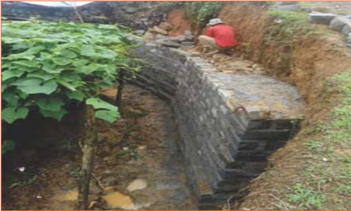
Figure 5: CRSM Retaining wall at NST Colony, Wokha
