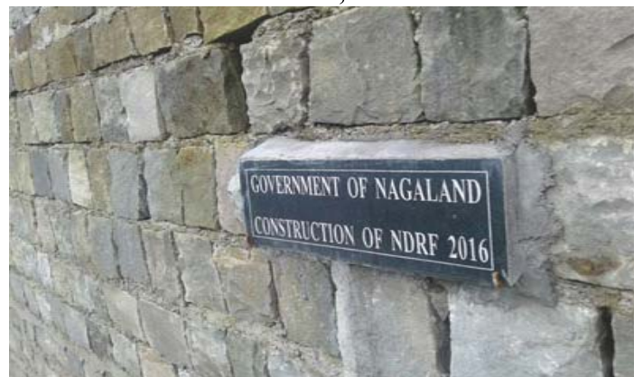
Figure 10: CRSM Retaining wall constructed by NDRF at Pfuchama, Kohima
