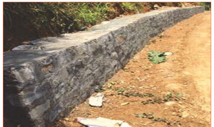
Figure 8 : CRSM Retaining wall at Wokha-Bokajan
