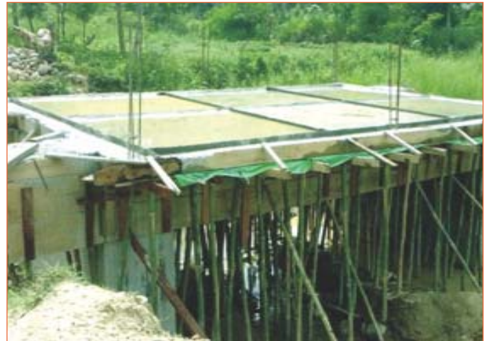
Figure 2: RCC Box Culvert at Chumukedima
