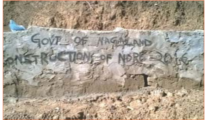
Figure 6 : CRSM Retaining wall at New Peren
