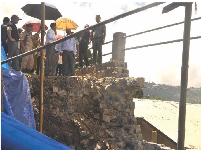
SITE INSPECTION AT DAKLANE KOHIMA
