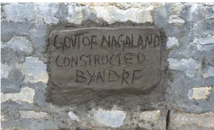
Figure 9: CRSM Retaining wall constructed by NDRF at Wokha-Bokajan Road Wokha-Bokajan Road
