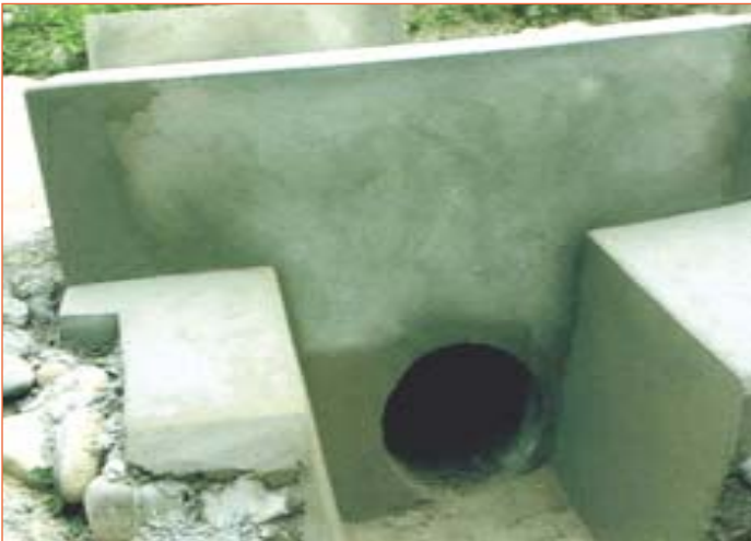
Figure 1: Hume pipe culvert at Chumukedima
