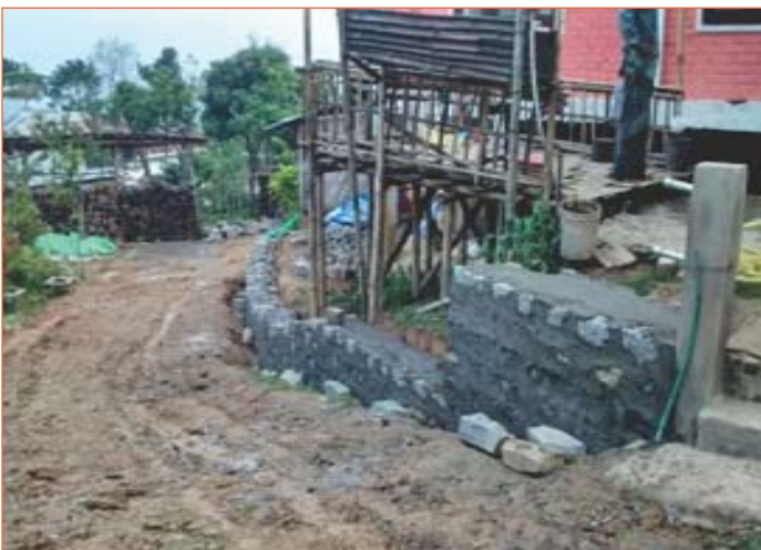
Figure 3: CRSM Retaining wall at Chungzia, Mokokchung
