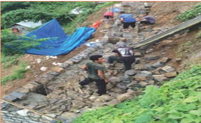
Figure 7 : RCC Composite Retaining wall at Lower AG, Kohima
